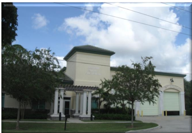
Fire Station 2610 SW 40th Ave. West Park, FL 33023
