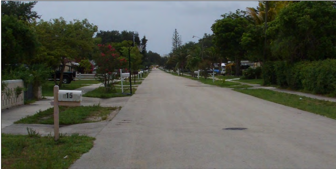
Most Local Streets have Continuous Sidewalks (Ronald Road)
