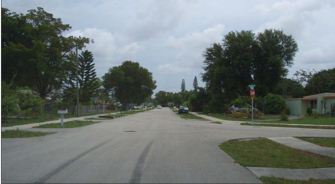
Wide Roads without Horizontal Breaks Can Promote High Speed Travel (SW 59 th Terrace)
