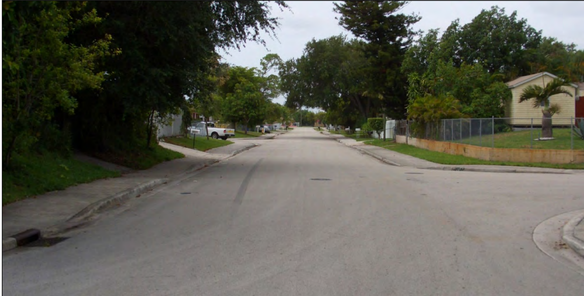
Curb and Gutter Section Along SW 58 th Avenue
